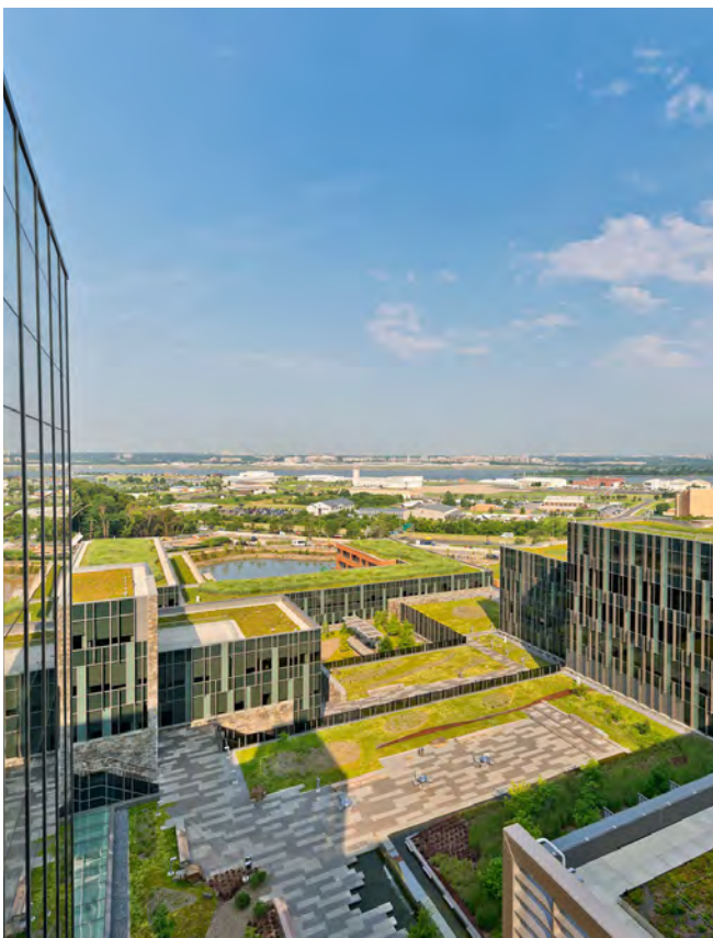
US Coast Guard Headquarters river view – a project by HOK. Photo courtesy of HOK.
