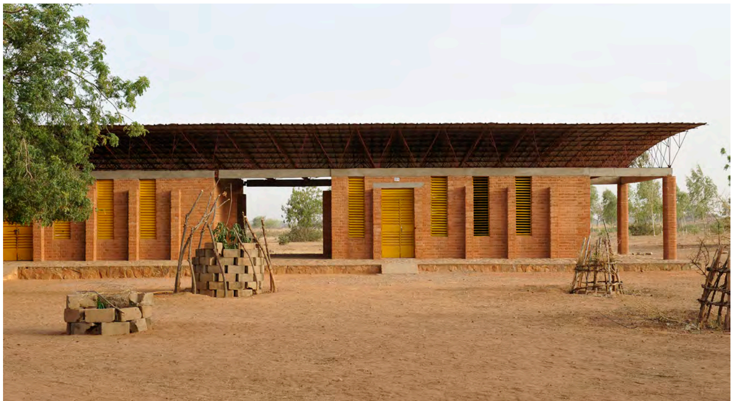
Gando Primary School. Photo courtesy of Erik-Jan Owerkerk and the Pritzker Architecture Prize.
